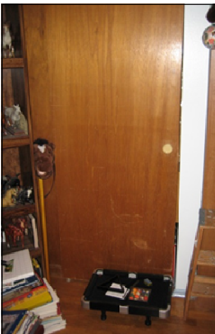
Figure 5: Closet door can still be shut.
